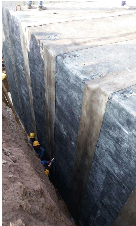
Extra Sealanting work on bottom
