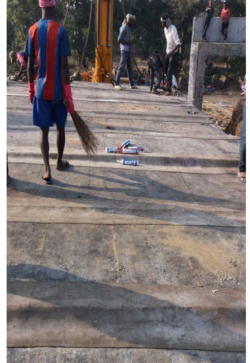
Laying of CC
