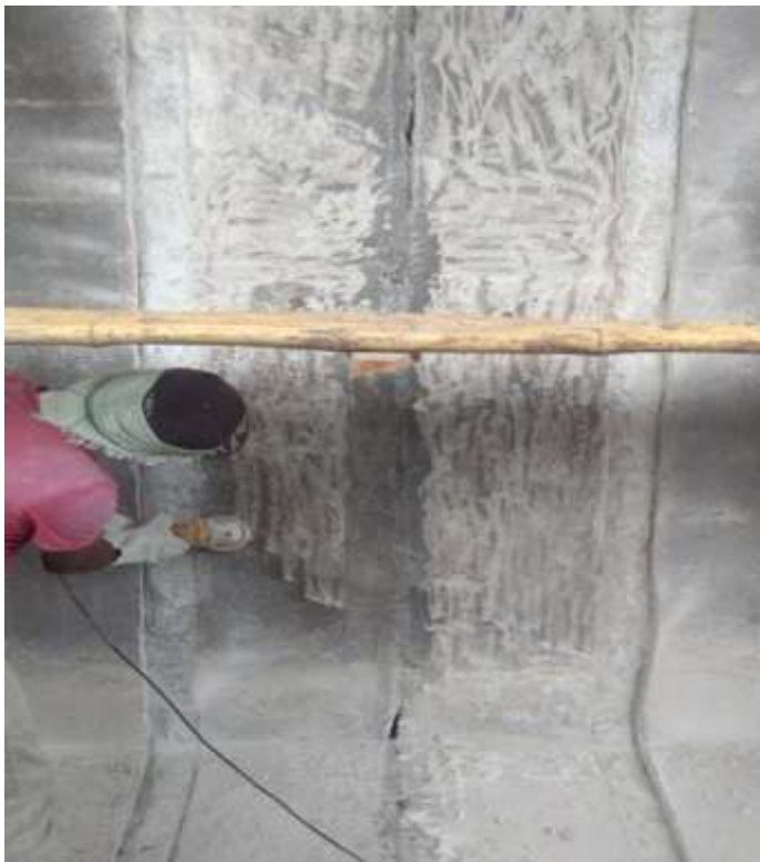
Cleaning & Dust removing
