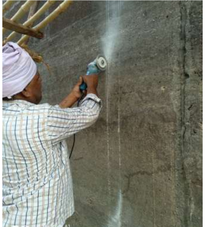
Concrete Cutting & Groove Formation
