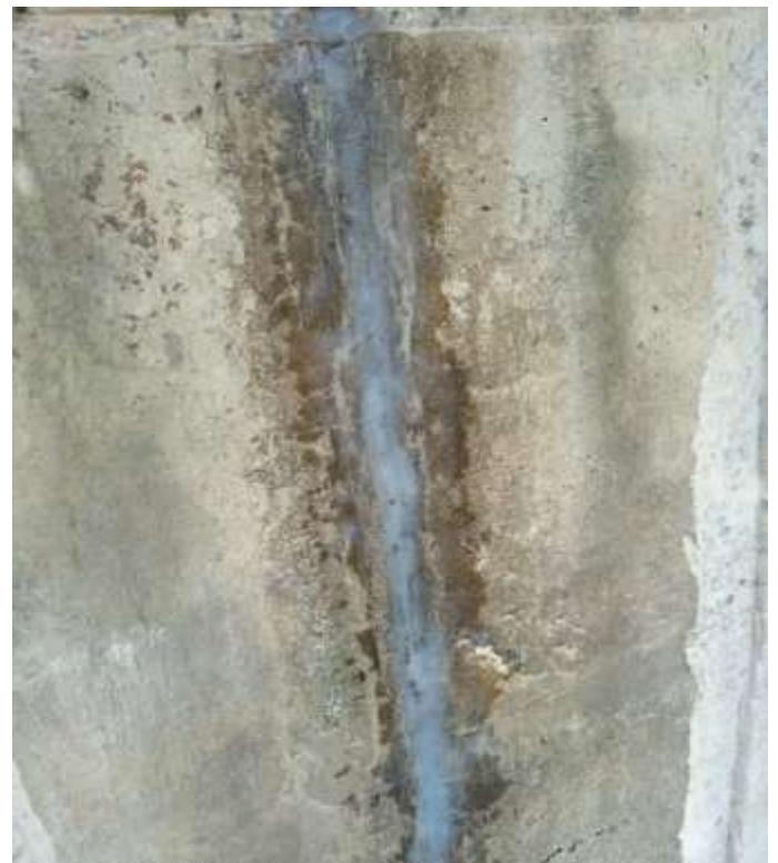
Filling Joints with Silicon Sealant
