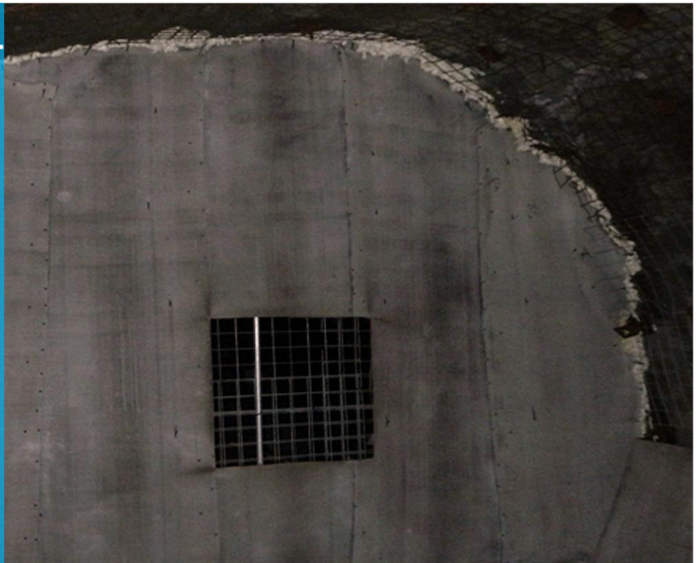
Completed Vent Wall
